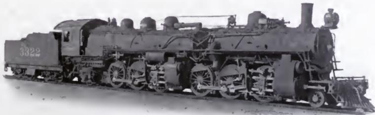
ARTICULATED LOCOMOTIVE WITH FLEXIBLE BOILER
